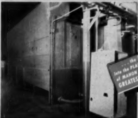
One of Four Mahon TYPE 54 AC-F PUMPLESS Hydro-Filter Spray Booths installed in the Porcelain Enamel Finishing Line of the same manufacturer referred to above. Note tubular sludge unloading conveyor casing at bottom of sludge tank.
